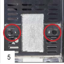
Tighten the screws (auto drilling) and make sure to align the holes.
